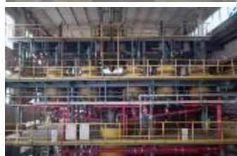
Resin color developer production workshop
