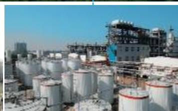
Raw material storage tanks
